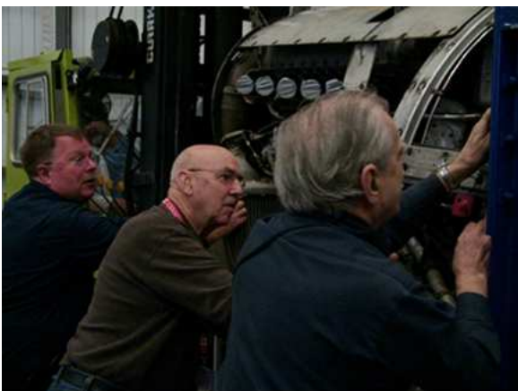
Figure 2: Nr 2 power plant removal. Bill Tate and Tim Timmins supervise the extraction of one of the four main attachment bolts from the mounting frame by Ted Devey.
