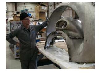
Figure 4: Murray Beauliau prepares to restore the lower front intake cowling: replace zeus fasteners, remove dents, repair corroded sections, polish...
